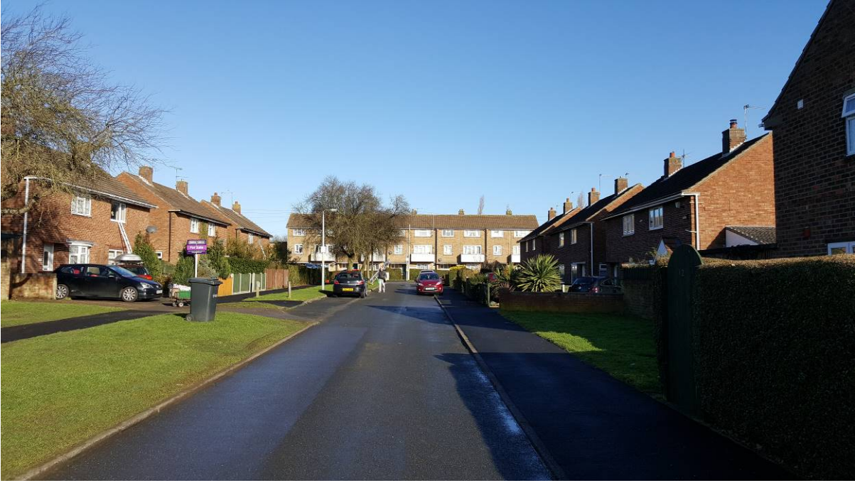
The view above is towards the end of Woodburn Close
