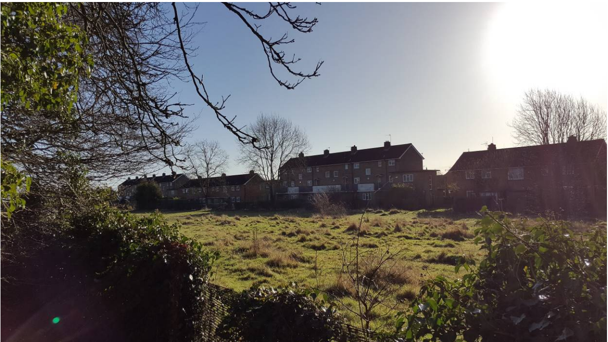
Above and below are views from the tree belt towards the three-storey buildings at the southern edge of the site
